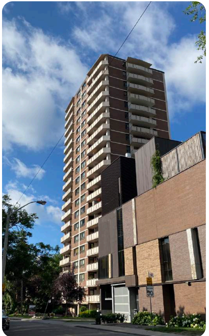
10 Huntley Street, looking southwest
