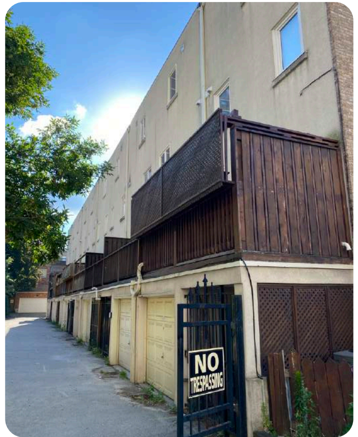
Parking garages and amenity terraces at 102 - 120 Earl Place (the subject site)
