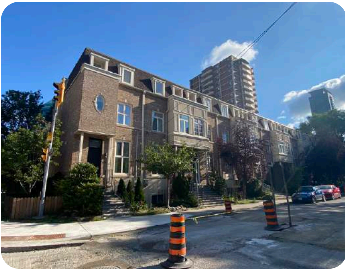
102 - 120 Earl Place (the subject site), looking northeast
