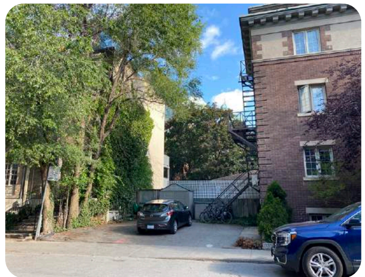
2 Earl Place, westerly side yard condition and surface parking spaces
