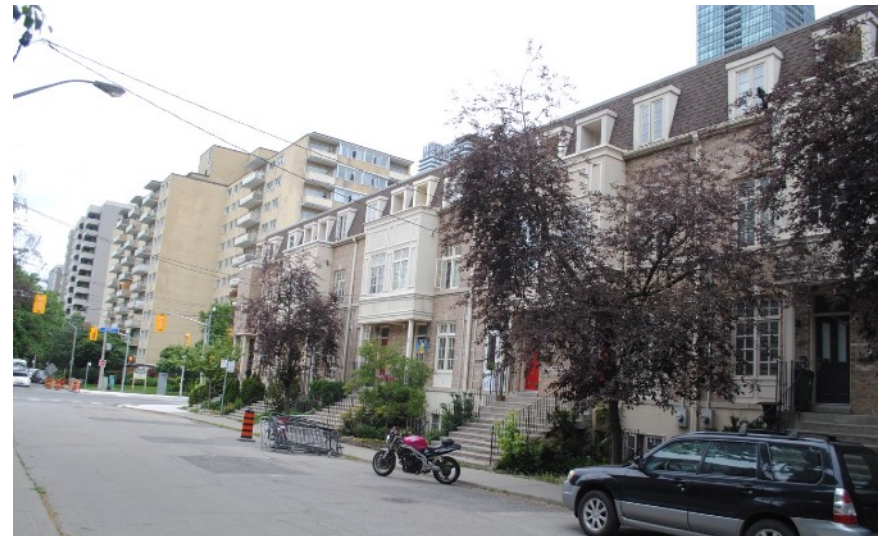
View towards the south side of the development site looking north-west from the south side of Earl Place. The row of 10-townhomes occupy more than 75% of the length of Earl Place, from Huntley to Jarvis Street.
