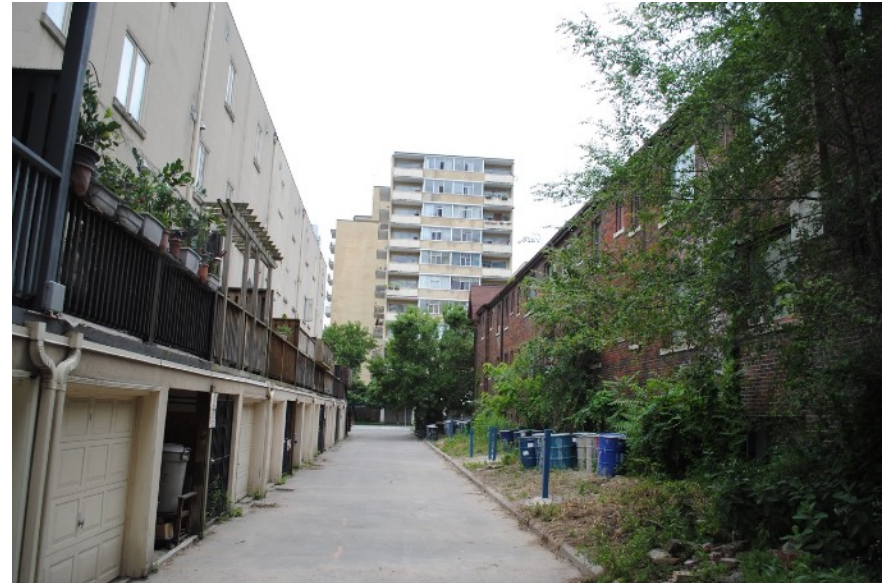
View from the eastern edge of the property, looking along the shared service lane for 102-120 Earl Place towards Jarvis Street. The 11-storey structure at 100 Gloucester(1958) is visible on the west side of Jarvis Street.
