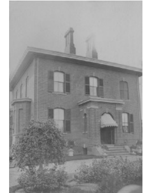
2) James Crowther house. Jarvis St., northwest corner of Gloucester St. 1881. (TPL)
