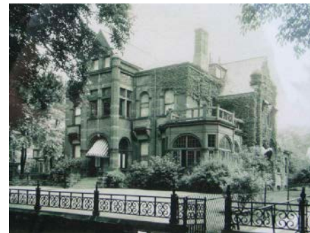
3) William R. Johnston House. 571 Jarvis Street, southeast corner Isabella Street. completed in 1875, and design by Langley, Langley, and Burke(TPL).
