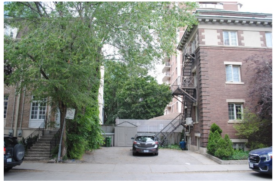
View of the Earl Apartments (1918), located on the northwest corner of Huntley Street and Earl Place. The subject site is located to the west, and is in-line with the adjacent heritage property.
