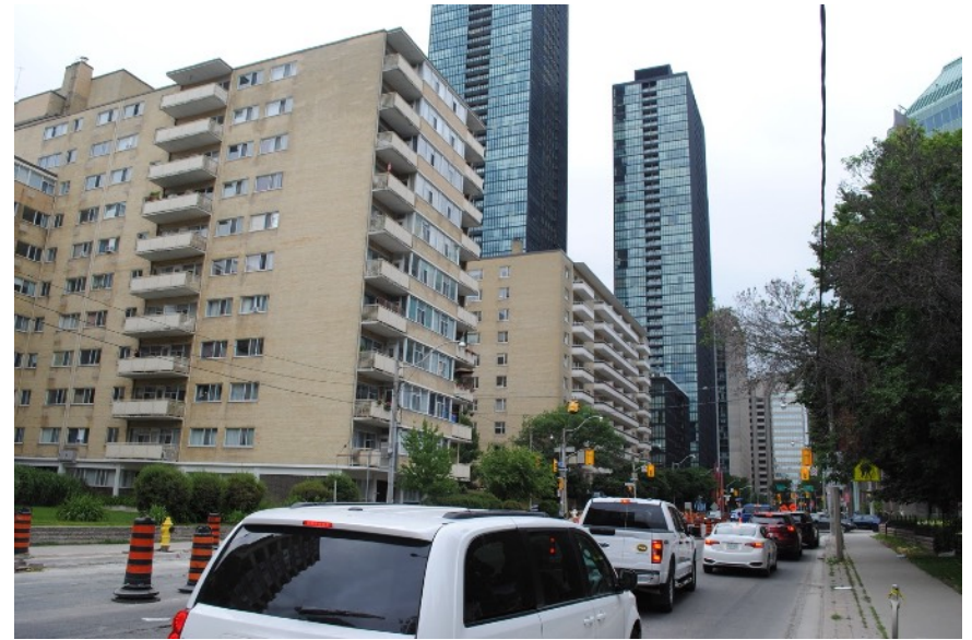
View from the development site looking northwest towards Bloor Street. The 11-storey buildings at 100 Gloucester / 105 Isabella (1958) with 99 Charles Street (2015), a 49-storey residential condominium known as 'X2'; 110 Charles Street east (2014) a 44-storey condominium known as 'X' visible in the background.
